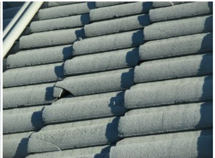
Many cracked and broken tiles on the roof. Recommend evaluation by a licensed roofing contractor.
