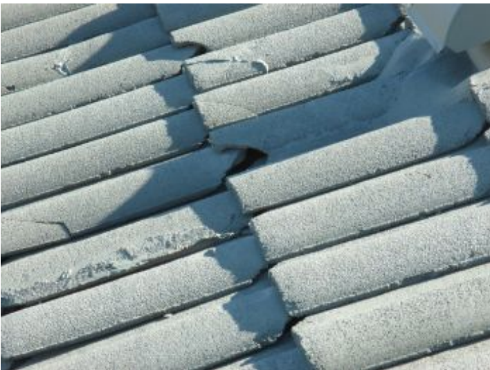
Many cracked and broken tiles on the roof. Recommend evaluation by a licensed roofing contractor.
