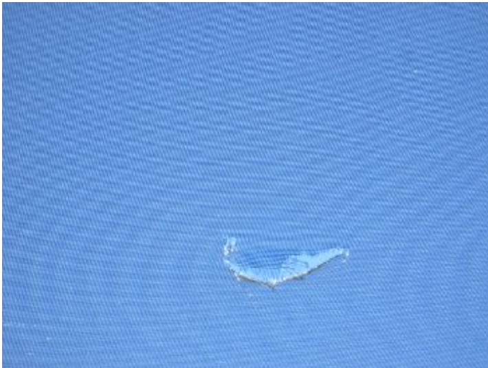
Torn/damaged screens.
